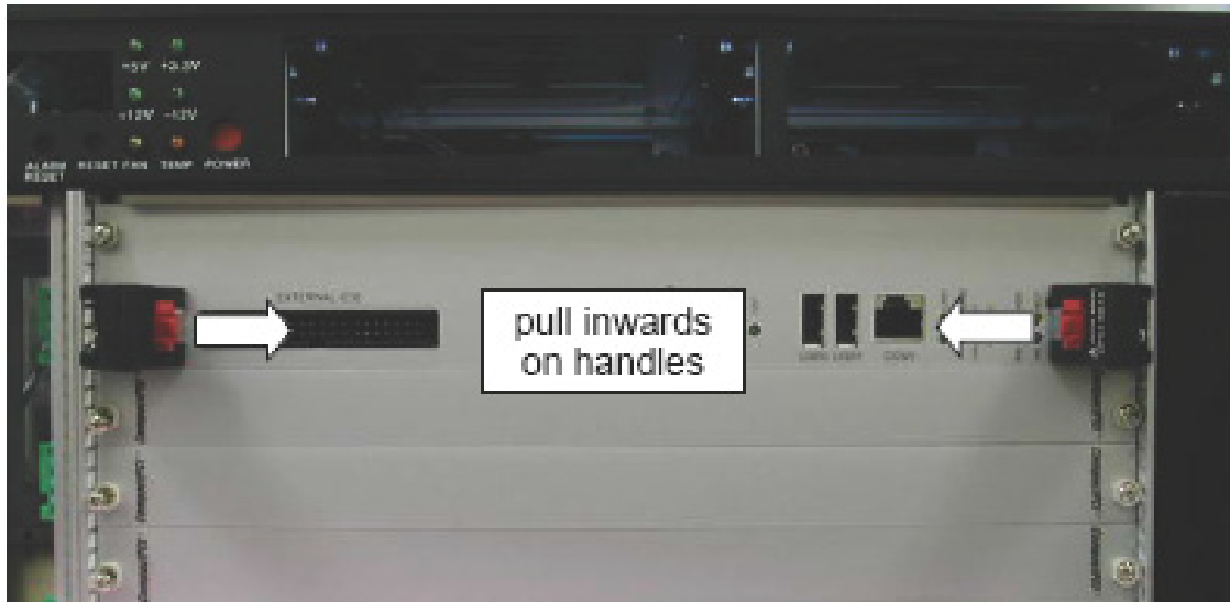
Figure 2-2: Latching the cPCI module handles securely.
