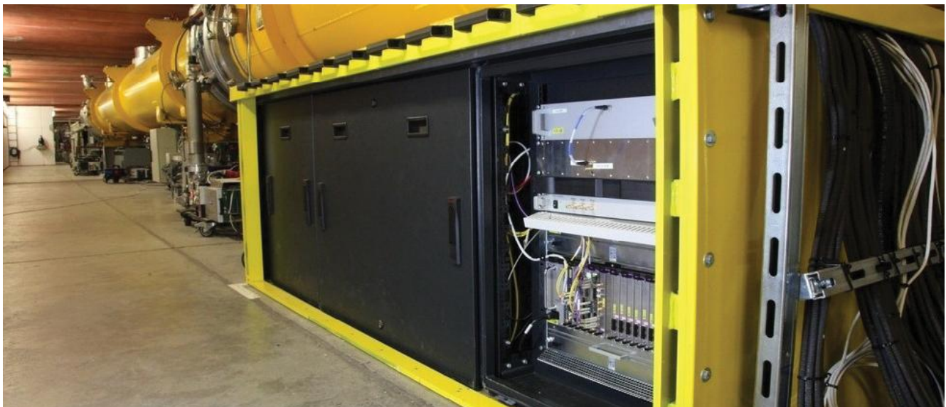
Fig.: Fully functional timing/LLRF control system based on MTCA.4 installed in FLASH (Free electron Laser in Hamburg). Generation of ultra-short laser pulses (4.1 nm).
